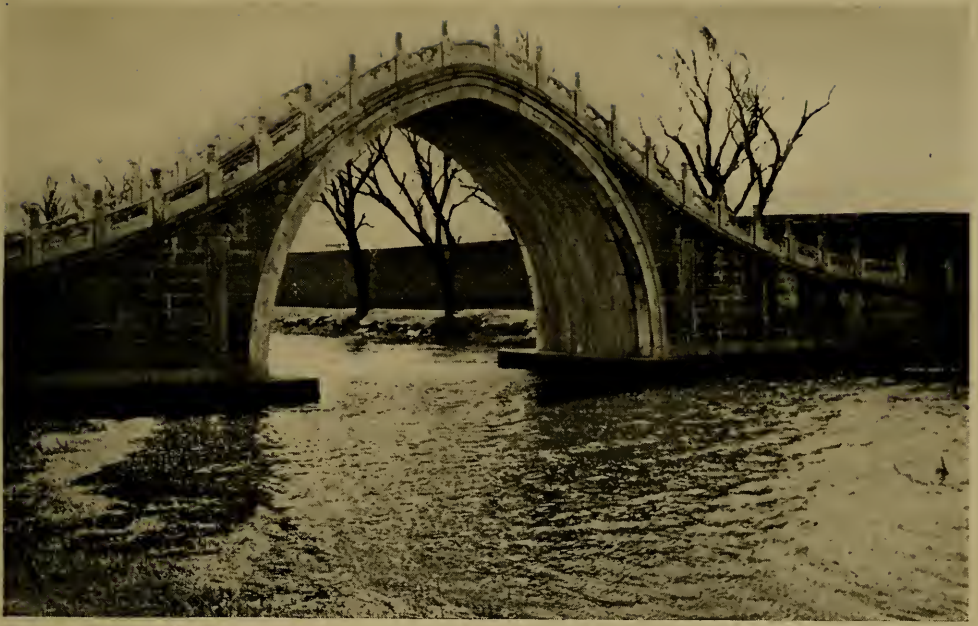
CAMEL'S BACK BRIDGE
